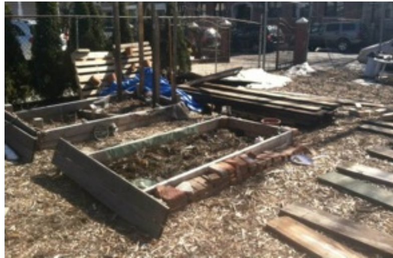
Building the plant beds.
